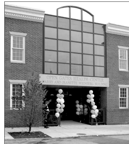
The new Open Gates facility on Washington Boulevard.
