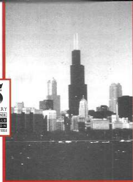
The 109-story Sears Tower—the largest private office complex in the world.
