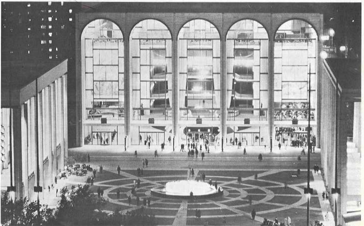
LINCOLN CENTER FOR THE PERFORMING ARTS. Lincoln Center's Metropolitan Opera House draws throngs of New Yorkers and visitors alike. Facade of the New York State Theater is visible at left, Avery Fisher Hall at right.
